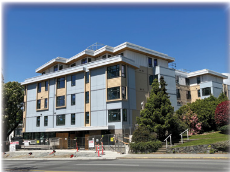
Cool Aid's new mixed-use development at 210 Gorge includes deeply subsidized and supported units, subsidized studio units, and near-market units.
